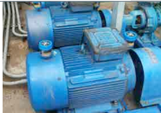
A combination of high-performance grease applied in a controlled manner via the Chesterton Lubri-Cup.
